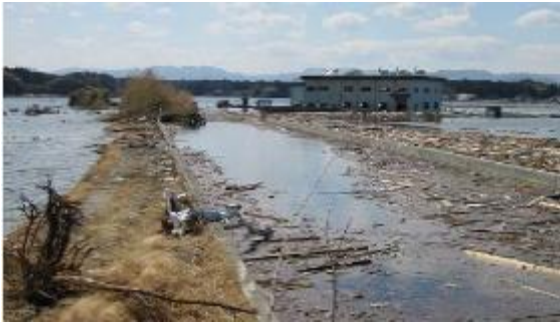
Tsunami-damaged drainage pump station and submerged farmland
